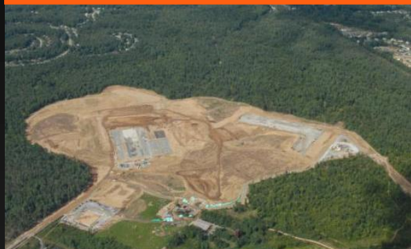
Malta site prior to GF construction
